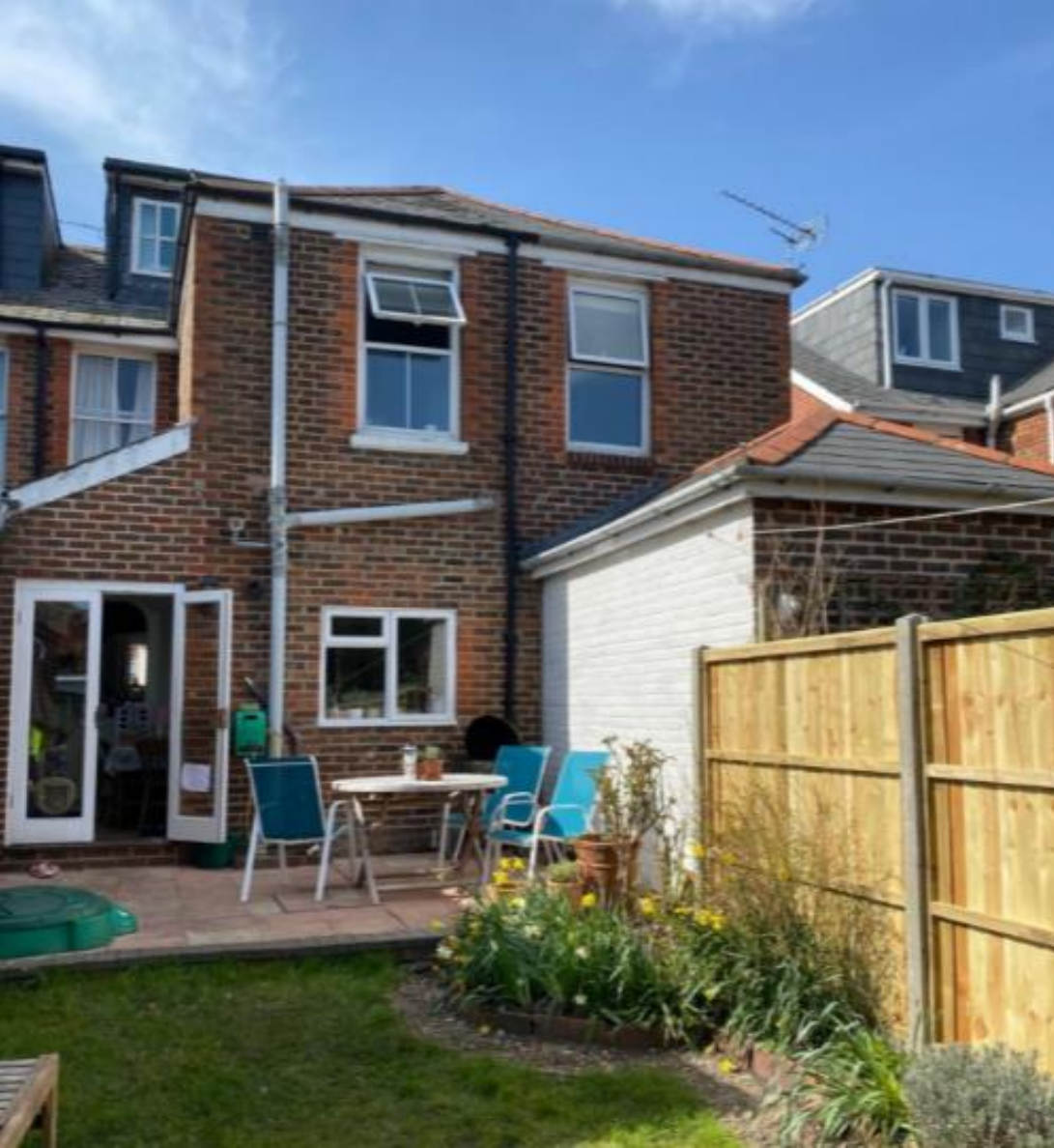
Neighbouring property to the north
